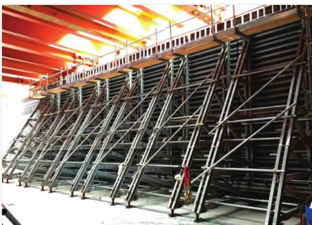
Tainan Underground Railway #C214 6.0M Single-Sided Wall Formwork
