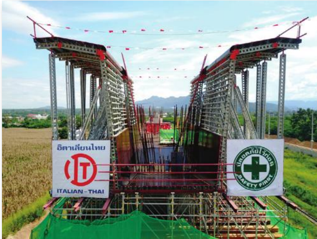
Central Taiwan Science Park - Frontage Road Bridge Formwork
