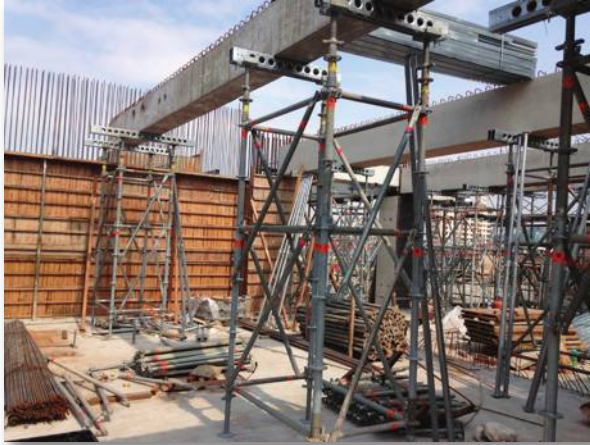
Top Beam as Main Bearer while shoring precast beams
