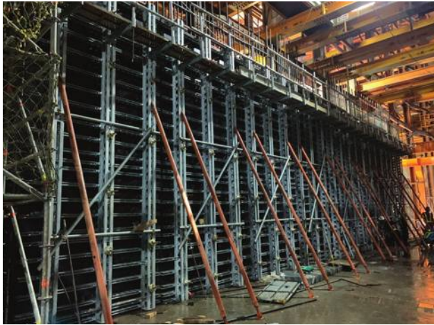
Taipei Metro WanDa Line 1st Phase CQ852 Compartment Wall 6M High Double-Sided Wall Formwork
