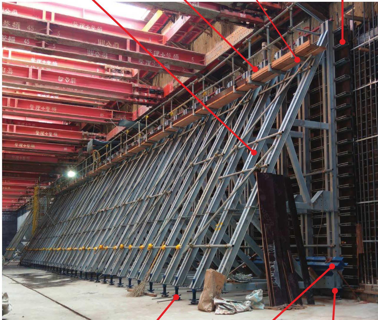
Junction plate of Back Jack Base & Universal Horn Jack Base
