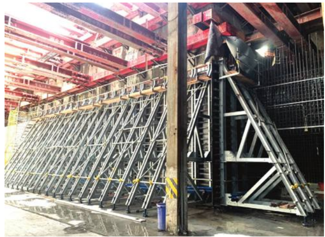
SUCOOT THAI – Pier Table Formwork & Shoring for Cantilever Method of Bridge Construction
