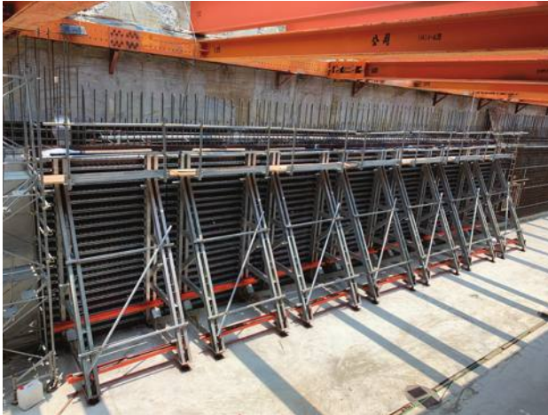
Kinmen Bridge - Pier Table (Box Girder H:7.5M) System Formwork & Access Tower
