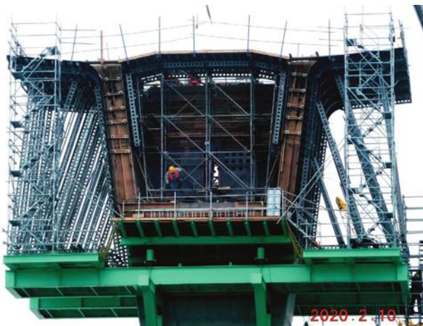
Ankeng Light Rail - Single-Sided Wall 1st Storey
