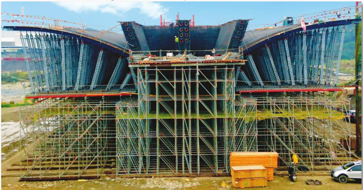
Top Beam connected with Base Beam as Second Bearer on an external formwork of superstructure of bridge formwork project
