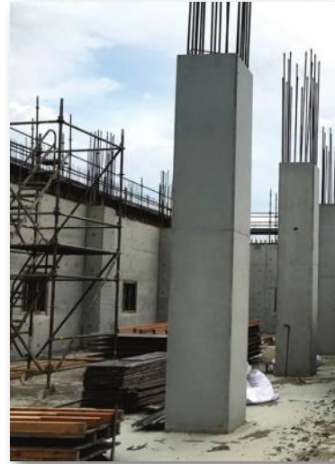
4.8M System Column Formwork (Finished)
