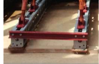
C-Channel 75x40x5x7mm
