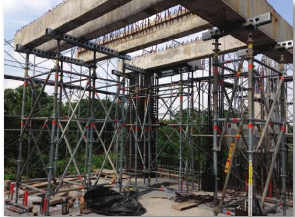
Top Beam as Main Bearer while shoring precast beams
