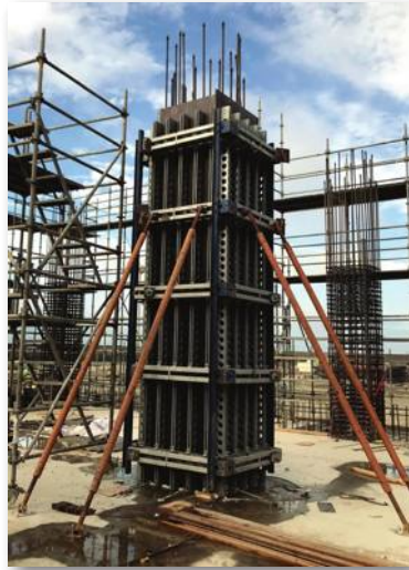
4.8M System Column Formwork (Under Construction)
