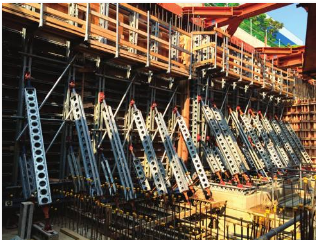
Taoyuan Longtan LY3 Basement 4.6M Single-Sided Wall Formwork
