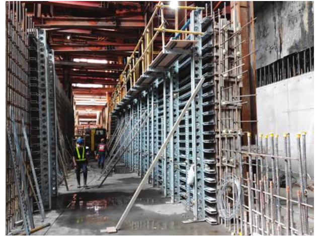
Taipei Metro WanDa Line 1st Phase CQ872 Compartment Wall 4.5M High Double- Sided Wall Formwork
