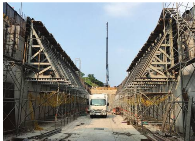
Ankeng Light Rail - Single-Sided Wall 2nd Storey
