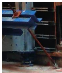
Pressing Beam+CONE-L + J Bolt
