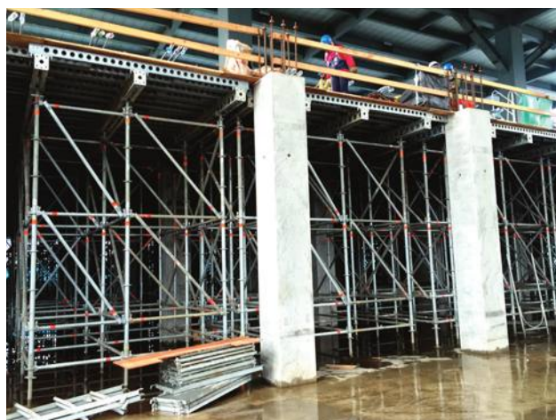
Taoyuan Longtan LY3 Factory Slab Formwork & Shoring
