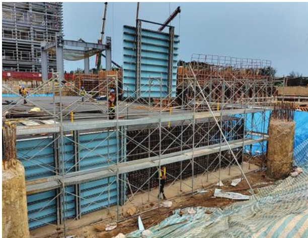
Datan Power Plant #7 STG Building 3.05M High Foundation Formwork
