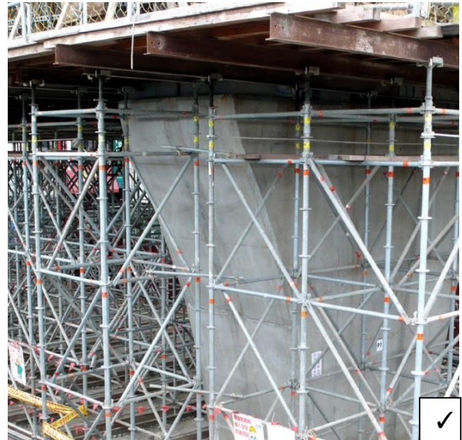
Assemble Horizontal on the top for reinforcement.
