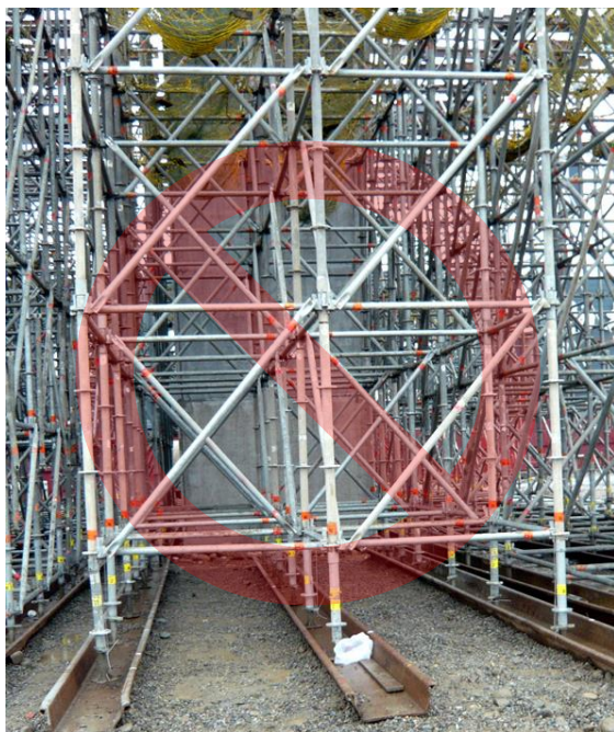
There are no Horizontal on the bottom.
