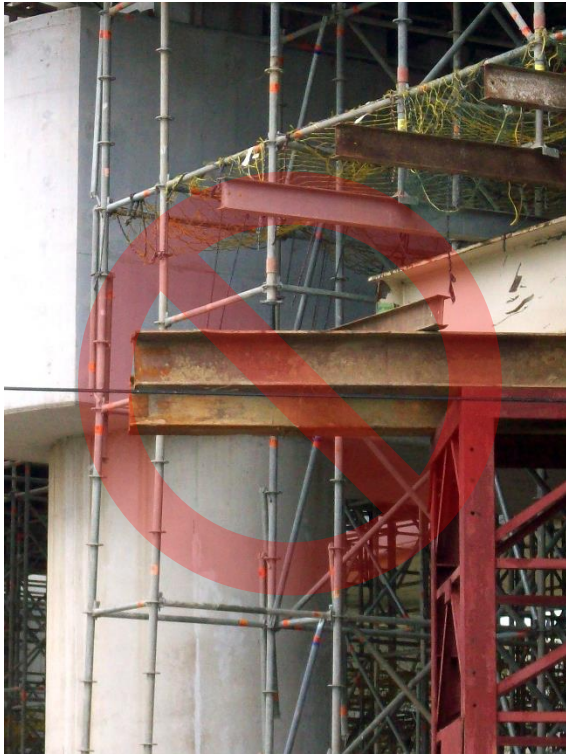
No assembly of Diagonal. The tower is crooked before Concrete pouring concrete.
