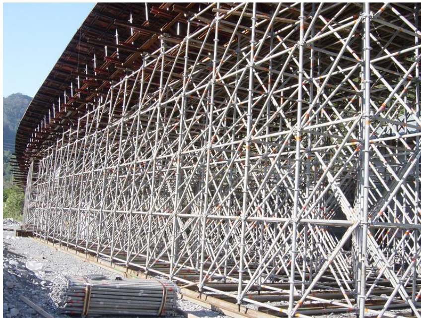
(7) Diagonal configuration in the same direction.
