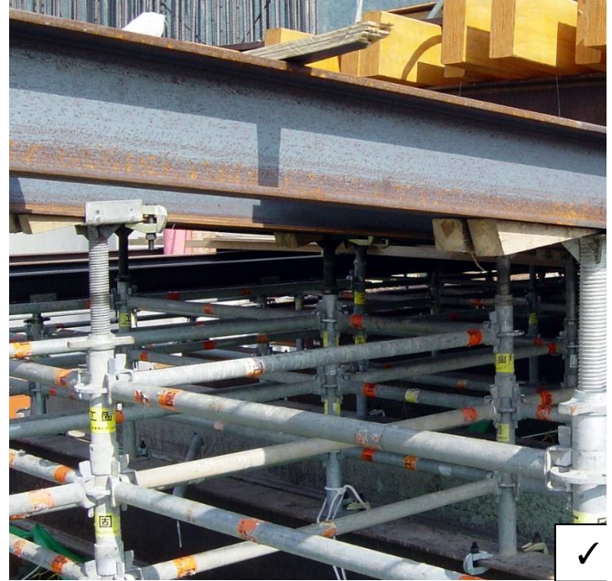
(13) Use the steel/wood wedge on the U-Head Jack
