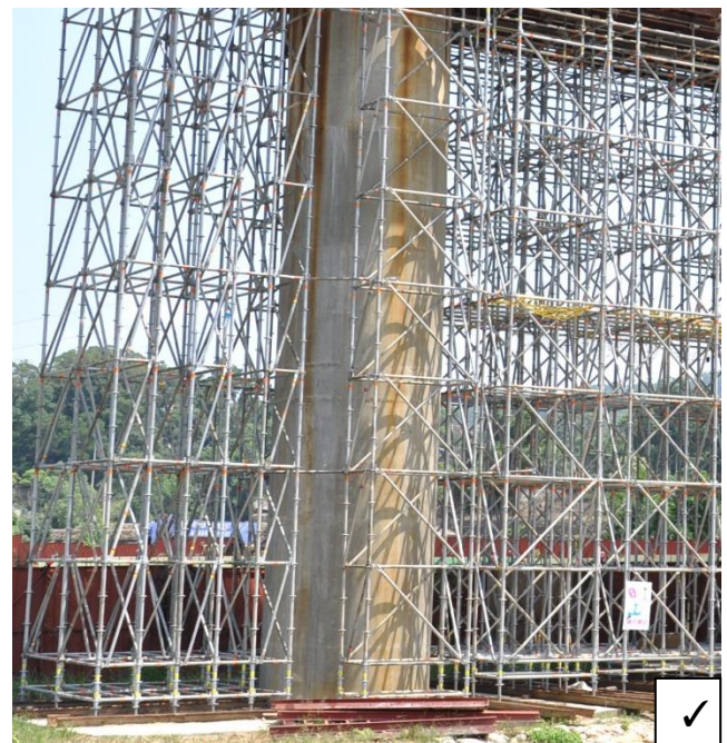
Assemble Horizontal on the bottom for reinforcement.
