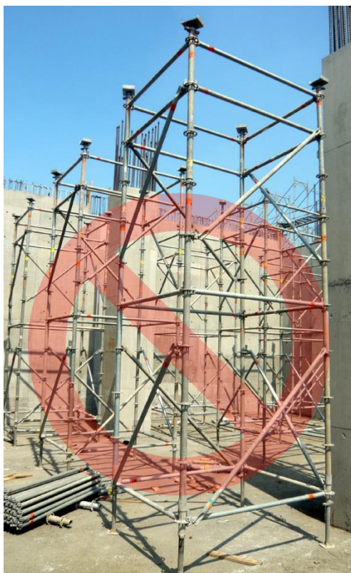
In order to save materials with the wrong assembly for 2 meter high.
