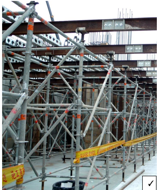
Assemble the Diagonal in every story.
