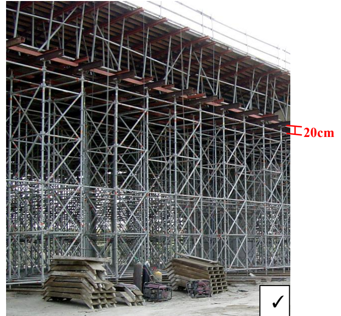
(9) Assembly of Horizontals on the top to make the cantilevered length shorter (less than 50cm).
