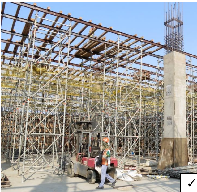
(10) Story Height: Less than 150cm, assemble Horizontals.
