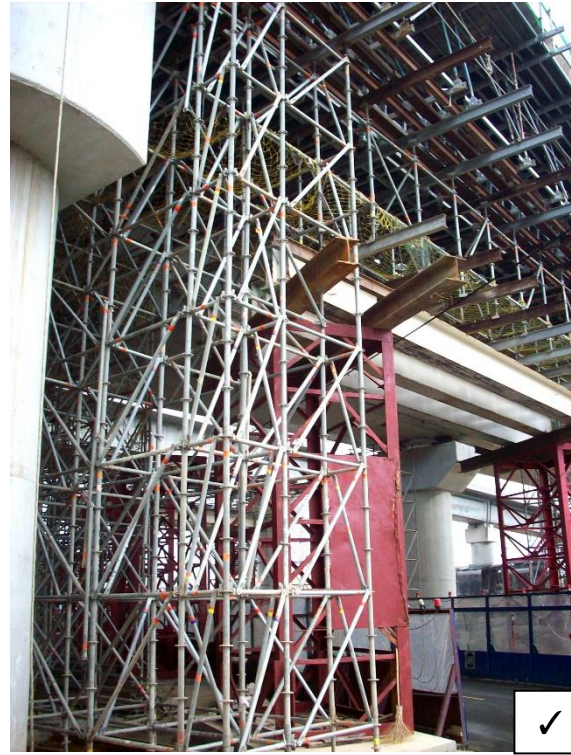
Assemble Diagonal for reinforcement.
