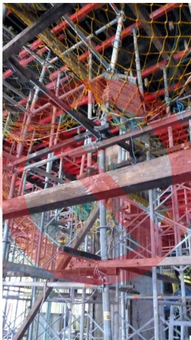
The factory construction without Diagonal, caused the bending after concrete pouring.
