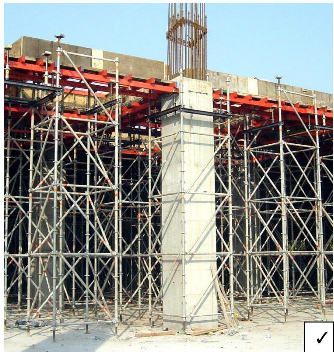
Assemble Diagonals in every story.
