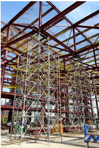
Taoyuan Convention and Exhibition Center – Shoring for Steel Structure Roof
