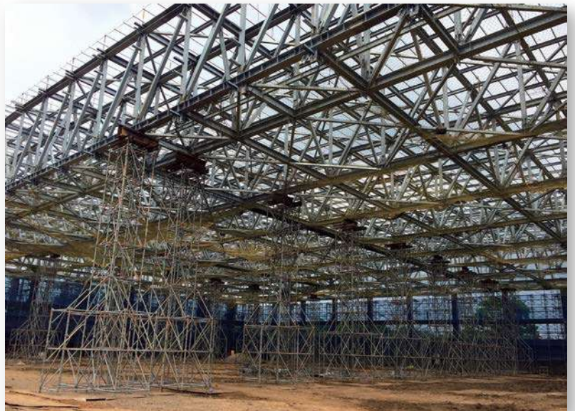
Shoring for Steel Structure Factory Assembly
