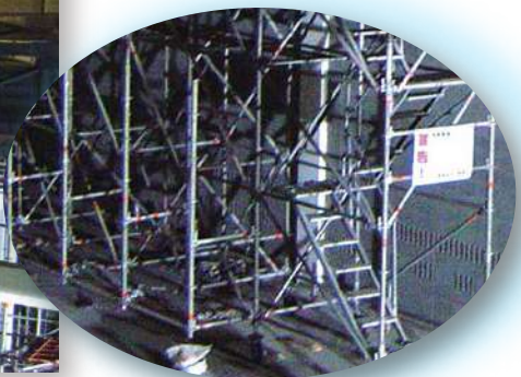
Access Scaffolding for High Level Installation Work
