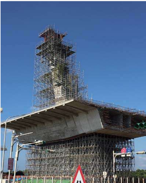
Cable-stayed Pylon - Pier Table Shoring
