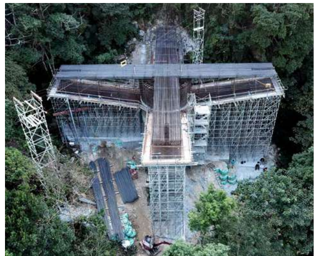
Taipower Tower Base Cross Beam Shoring
