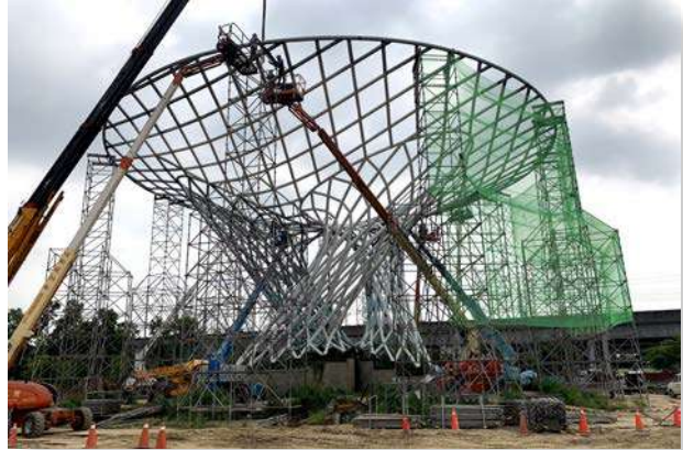
Thailand MRT Station – Shoring for Precast Beam
