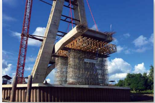
Indonesia Bridge Pylon Shoring
