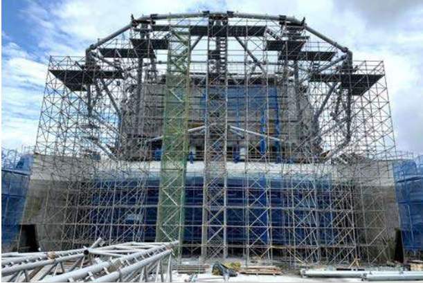
Taoyuan Convention and Exhibition Center – Shoring for Steel Structure Roof
