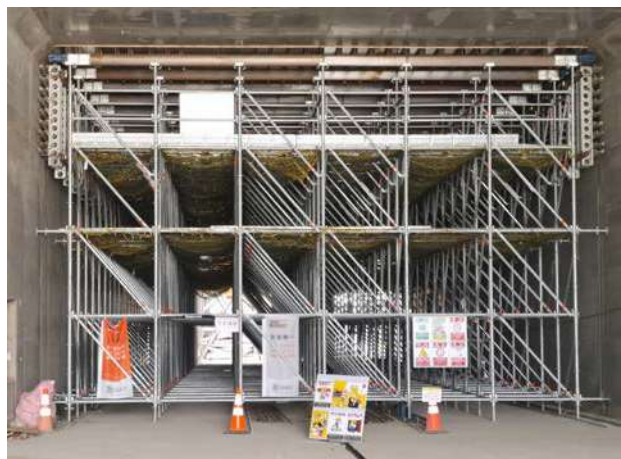
Underground Railway, Cut-and-cover Tunnel Slab Formwork and Shoring
