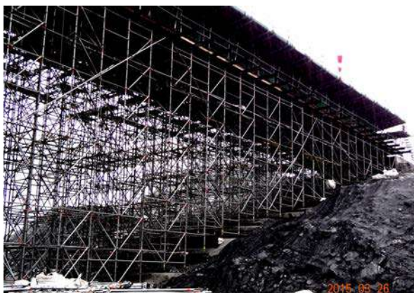
Superstructure Shoring in Slope
