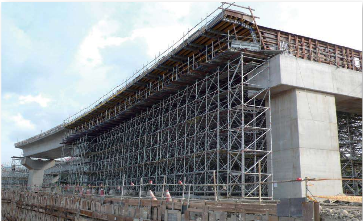
Taipei MRT- Superstructure Formwork and Shoring
