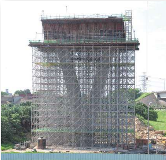
Y-Shaped Pier Cap Shoring
