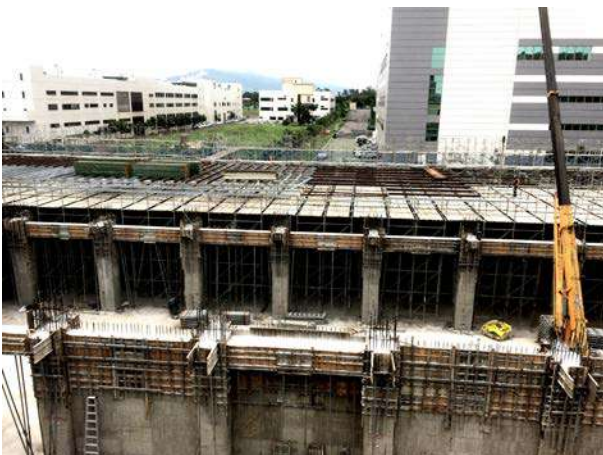
Hi-Tech Factory Slab Shoring
