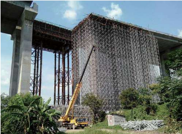
Chongqing, China H:37m Bridge Shoring
