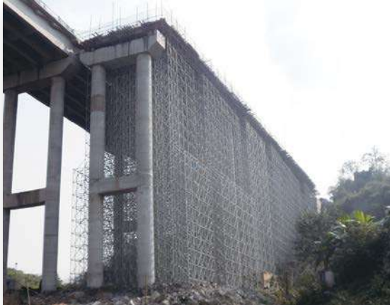
China Chongqing Bridge Three-span Shoring(6-30m height)
