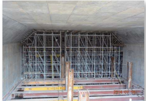
Underground, Cut-and-cover Tunnel Slab Shoring
