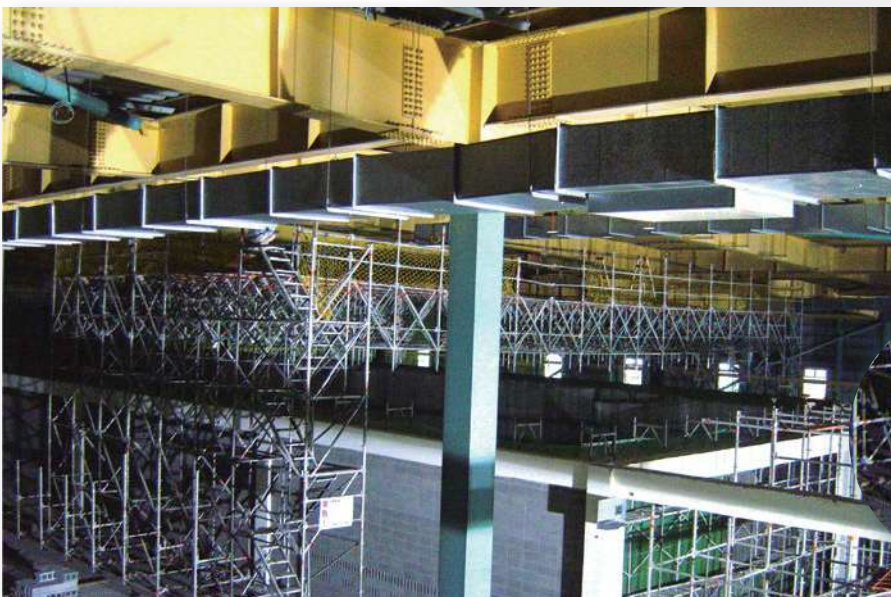
Access Scaffolding for High Level Installation Work
