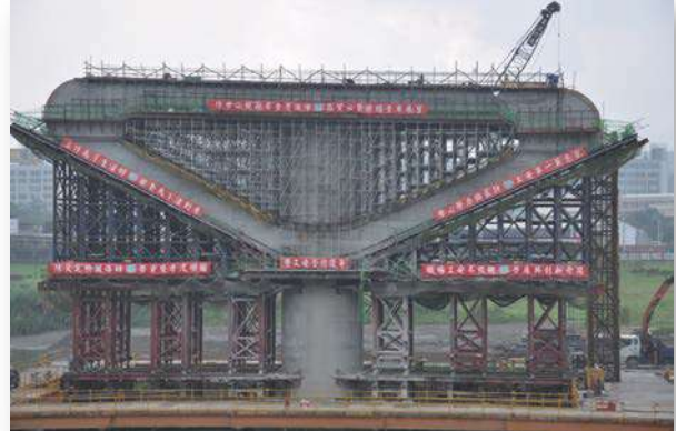
Taipei MRT- Superstructure Formwork and Shoring
