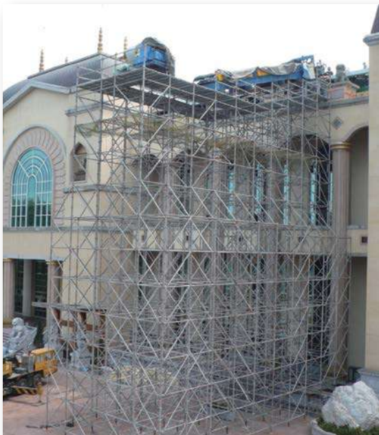
Shoring Platform for Roof Forming Machine
