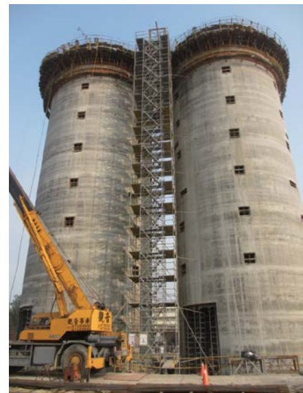
Staircase for Slip Form
