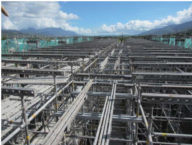
Slab Shoring for Power Station
