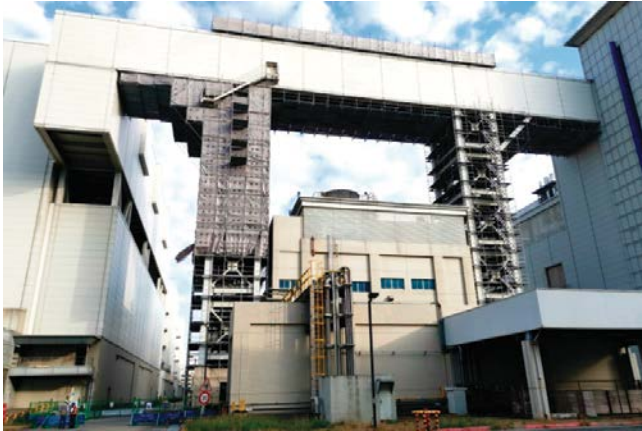
Suspended Scaffolding (36m Height)
